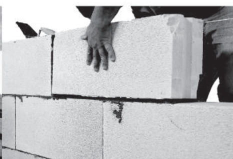
Light-weight Block Laying
