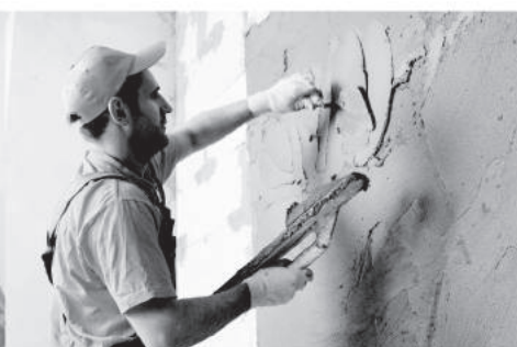
Light-weight block plastering
