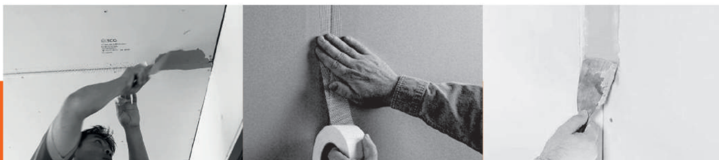
Jointing Fiber Cement Board
